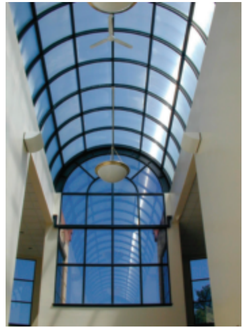
Yeshiva of Spring Valley, Spring Valley NY Glazing Contractor: Ailamos, Bronx NY
